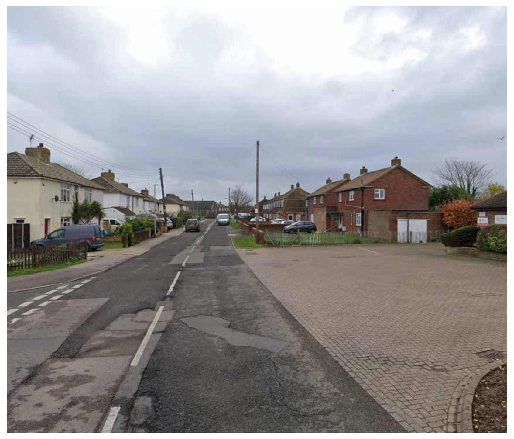
7. View along Chapel Road
