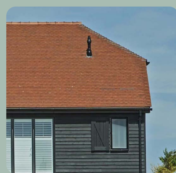
Half-hipped barn style roof
