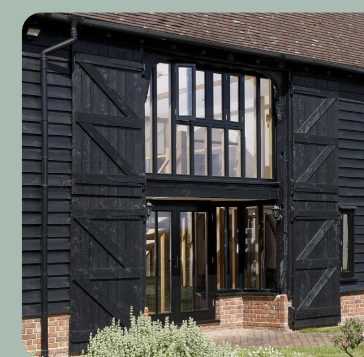
Large barn-style windows
