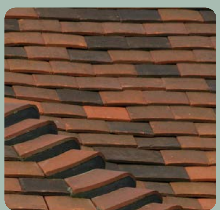
Clay tile roofing
