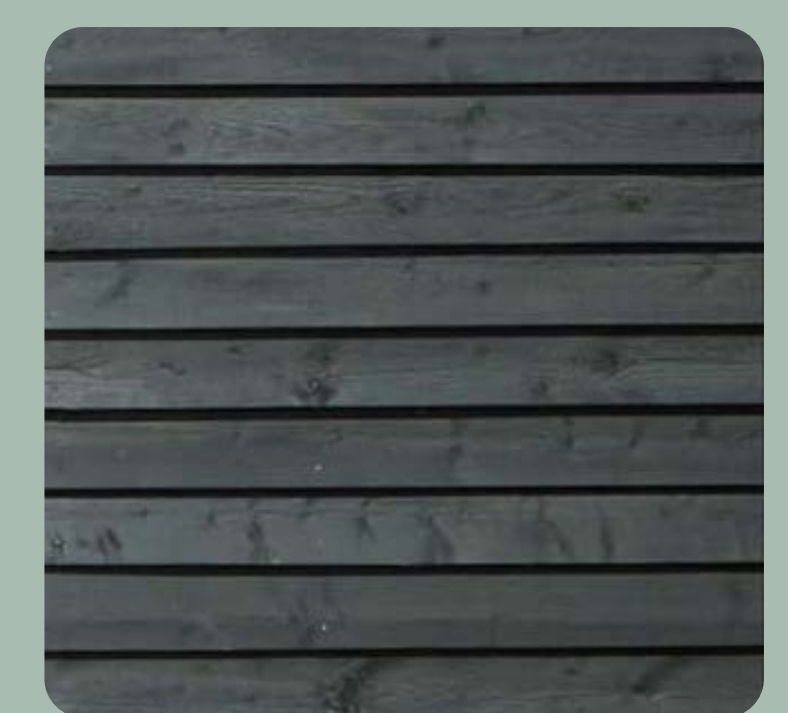
Black timber weatherboarding
