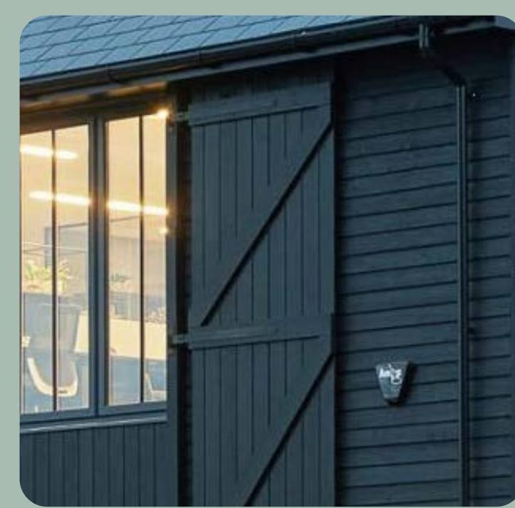
Black timber shutters
